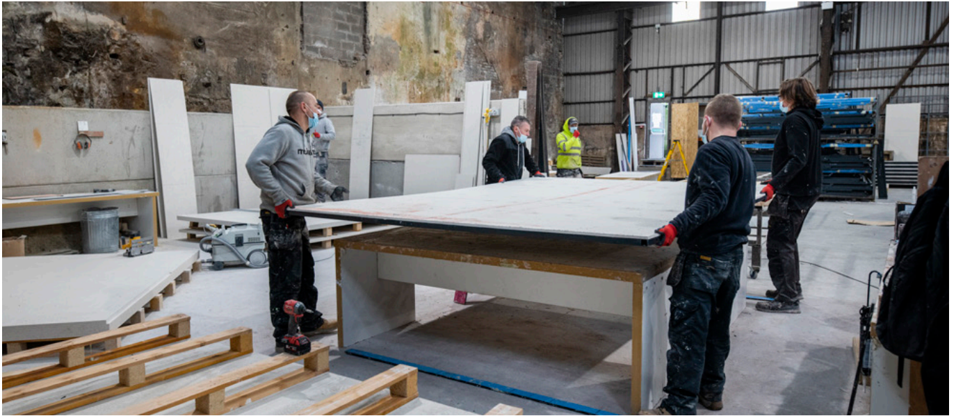
↑ 1. First stage of construction.
